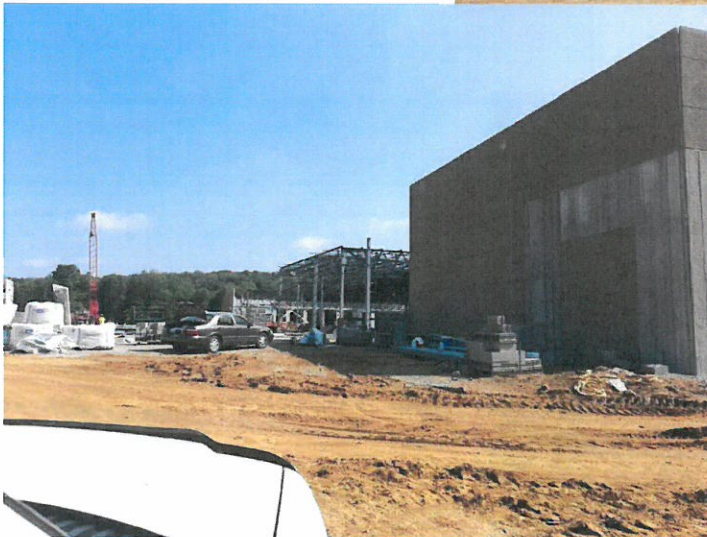
Wal-Mart Supercenter under construction
