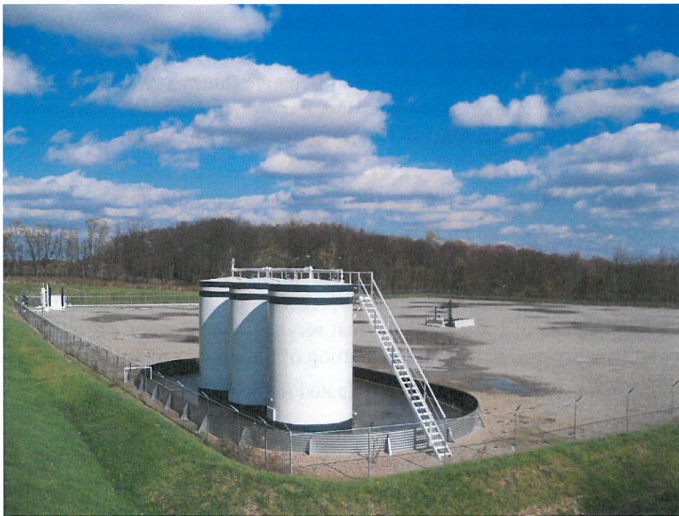
Picture of a completed well site
