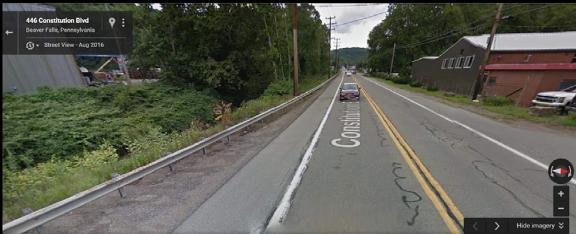
17 - SR 51 at Red Building looking west
