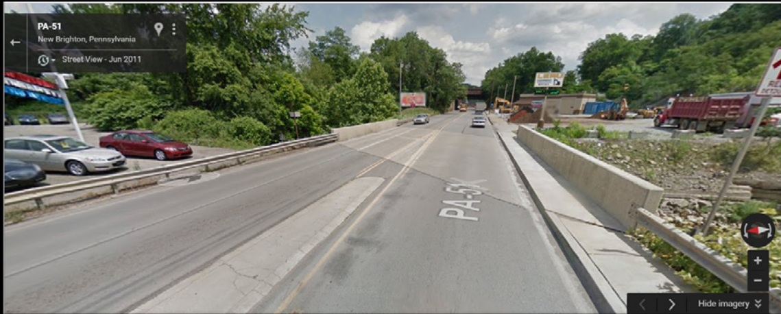
8 - SR 51 Bridge - west of LERU Equipment
