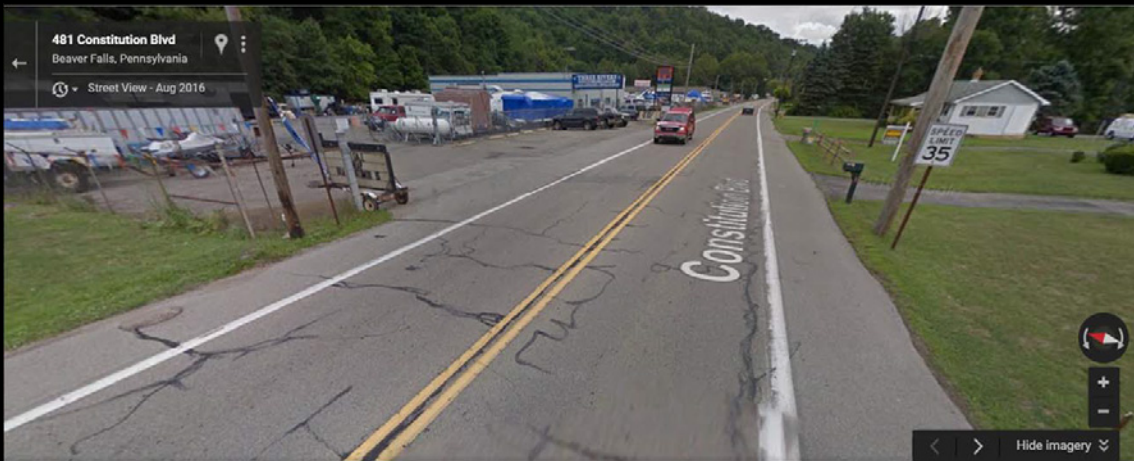
19 - SR 51 at Blakes Mini-Storage looking east
