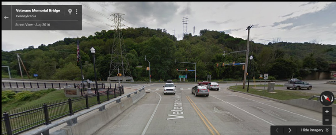
3 - Veterans Bridge - North
