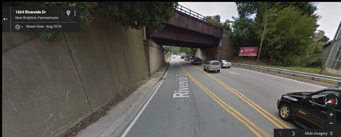
6 - SR 51 at Railroad Overpass
