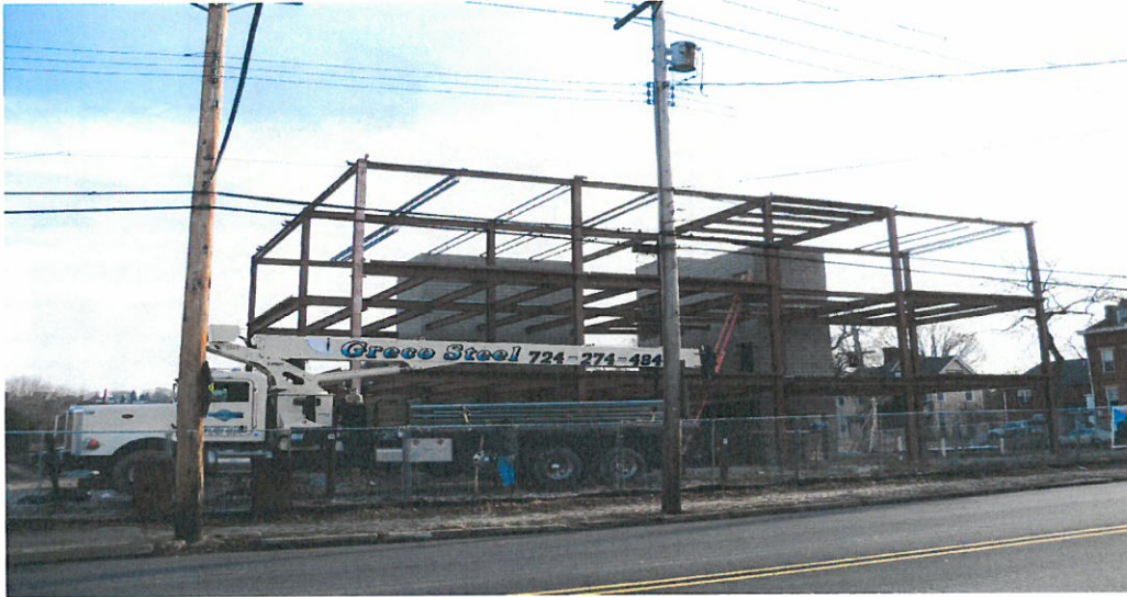
Trinity Office Building (under construction) Beaver Borough
