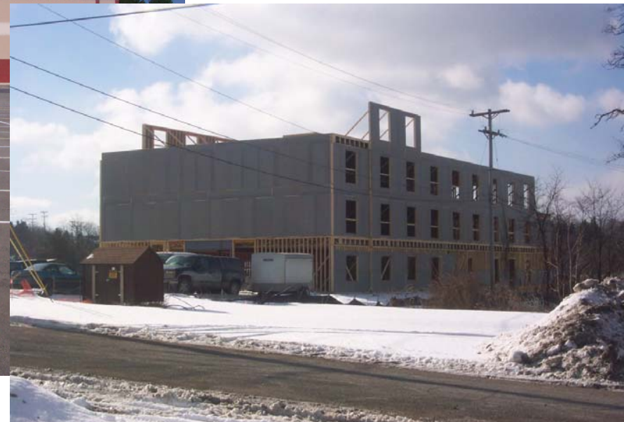
Hampton Inn under construction
