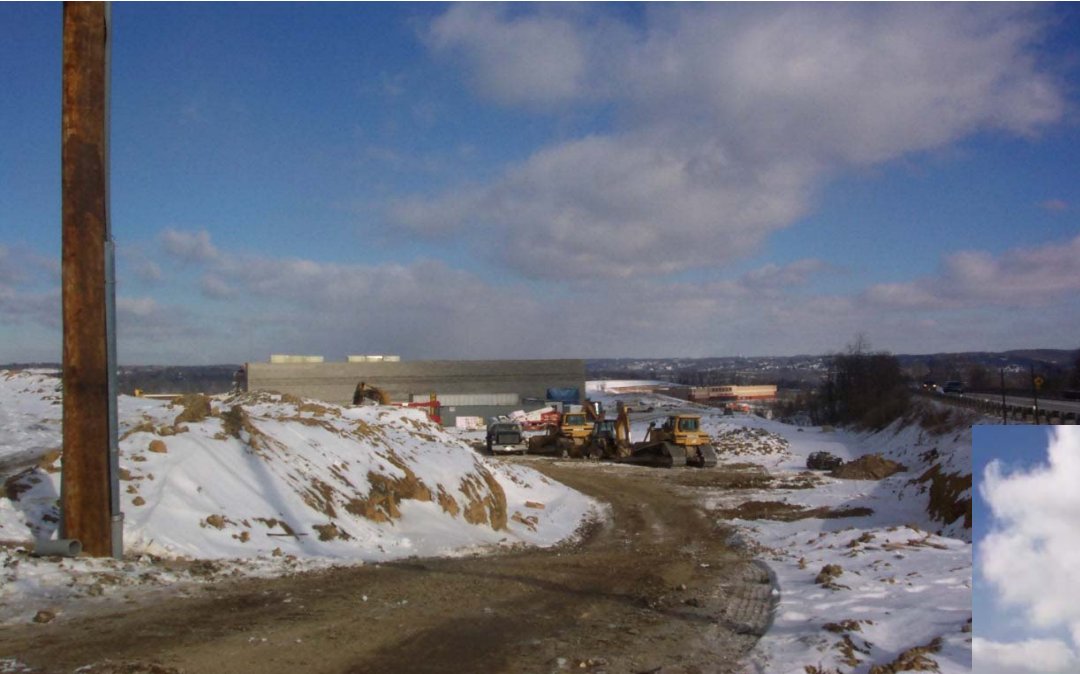
Best Buy under construction
