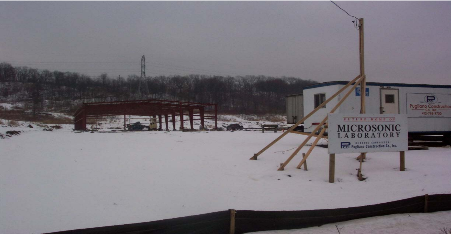
Microsonic Laboratory under construction
