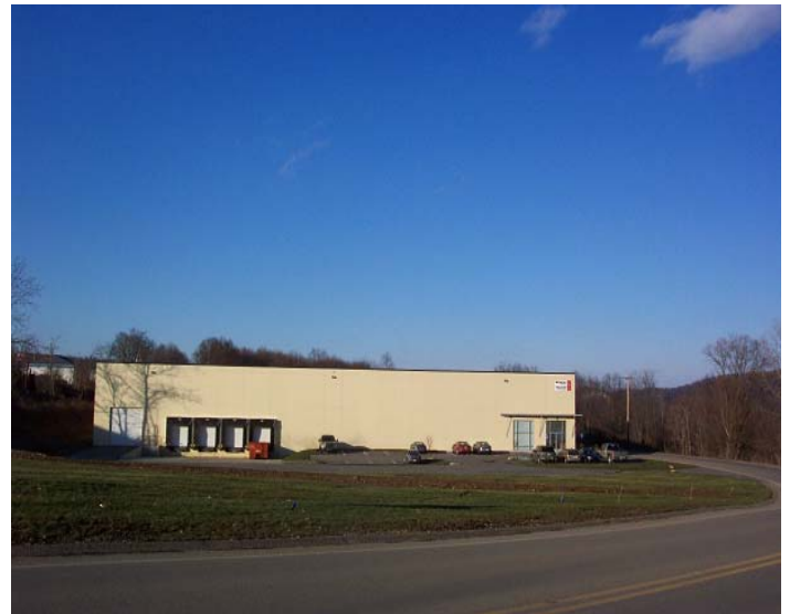
Westgate Business Park Phase II
