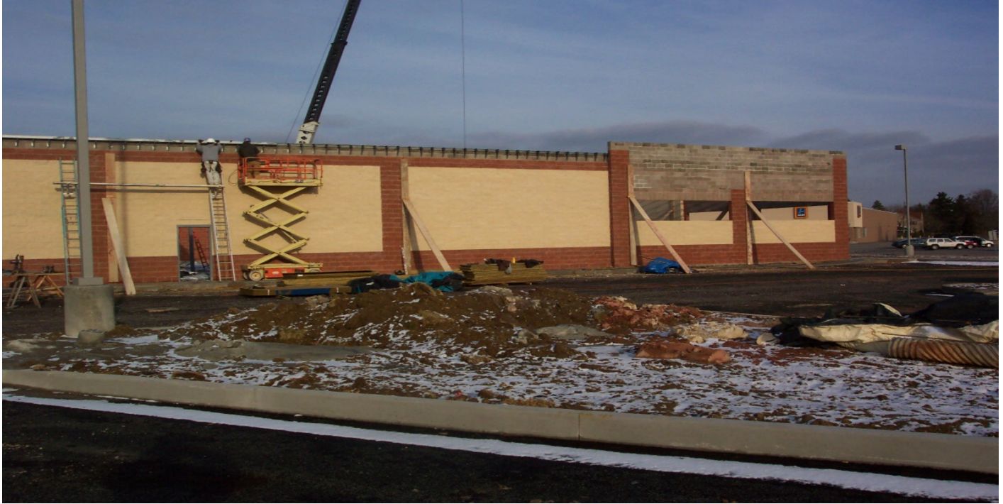
Chippewa CVS # 4162 (Under Construction)
