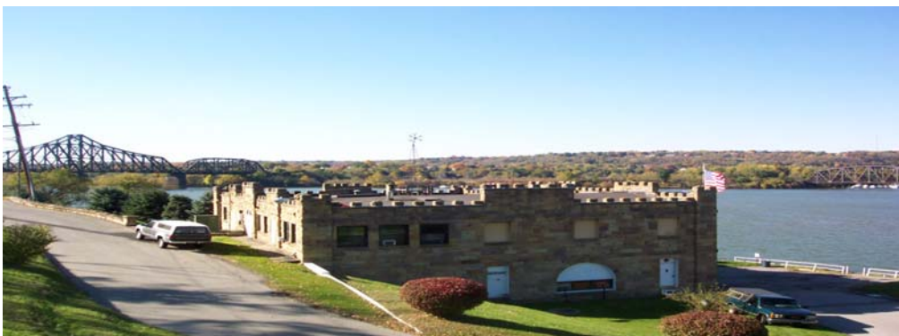
Photograph above is the Borough of Monaca Municipal Authority water intake facility , Beaver County
