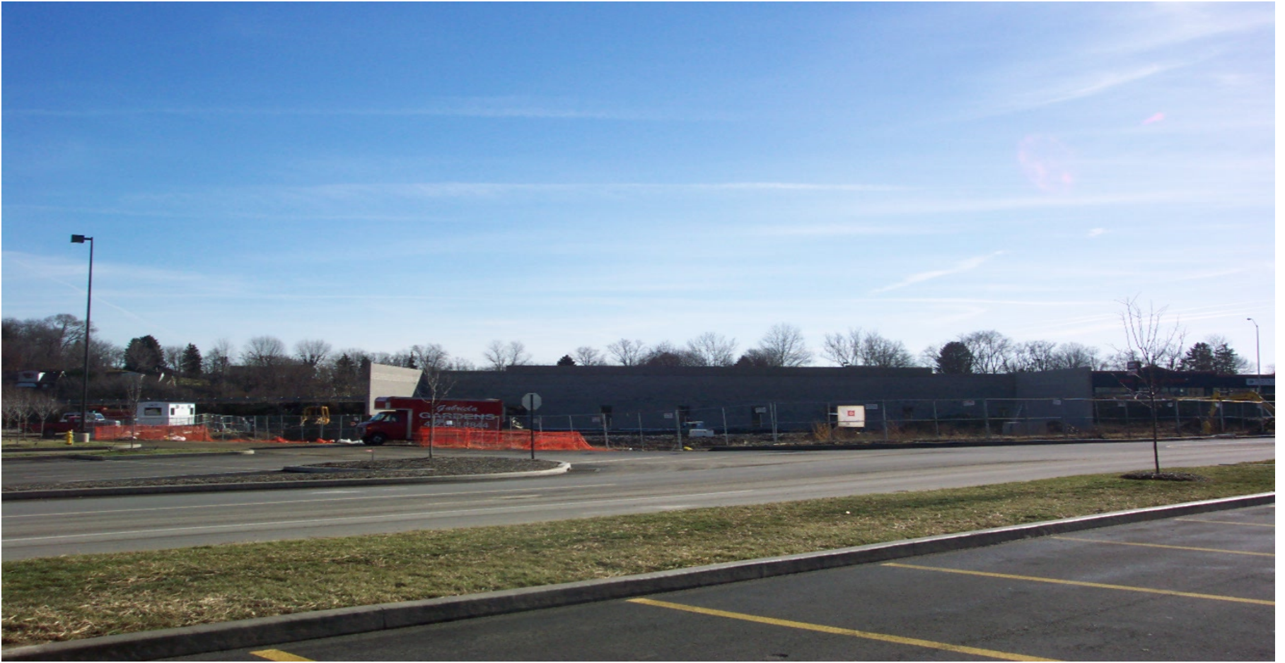
Center Point Shopping Center LD under construction
