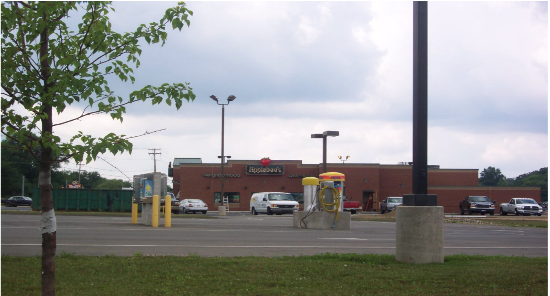
Completed Applebee's Chippewa
