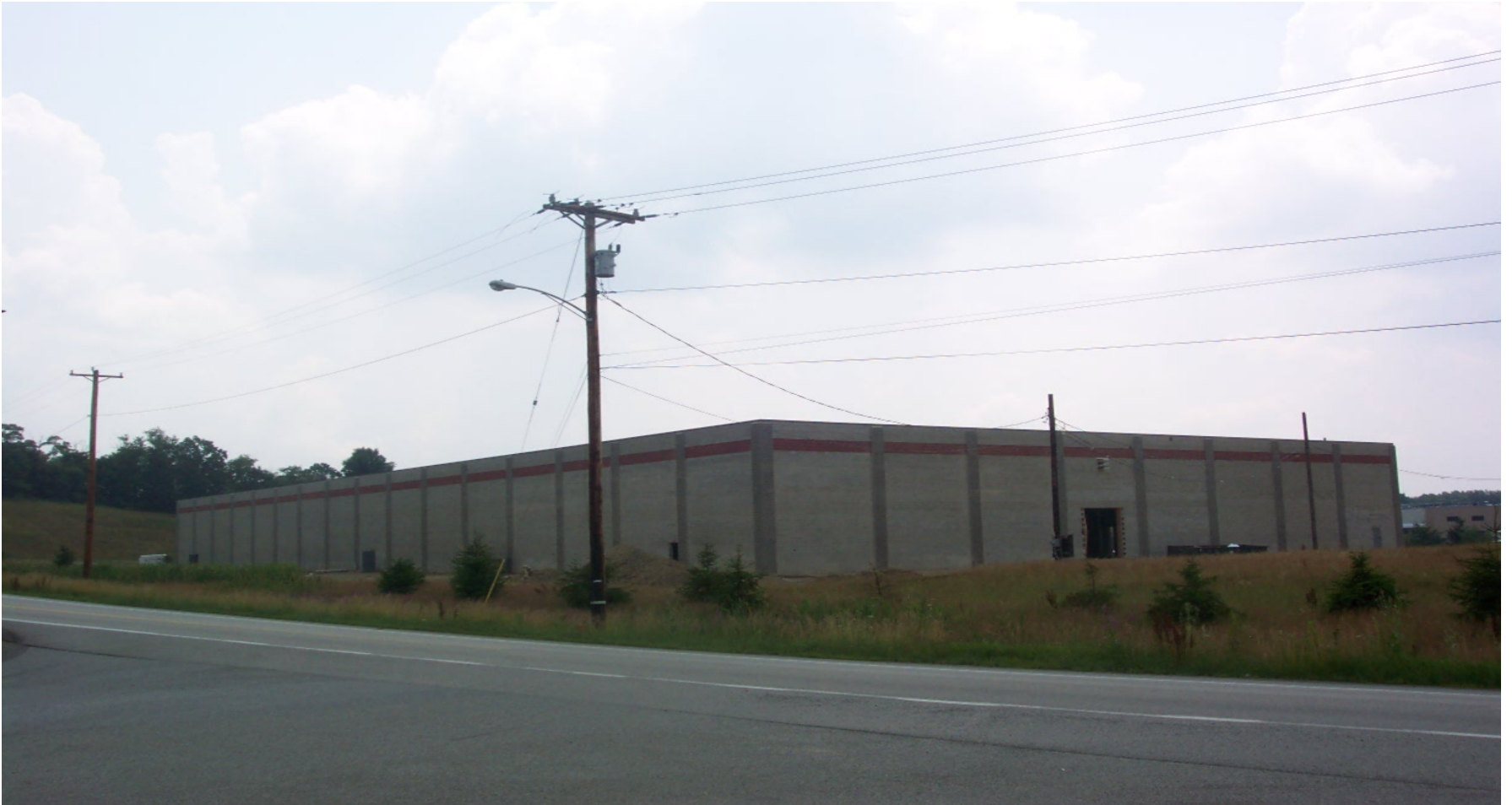
Tri County Commerce Park Phase 5, Building 5 completed
