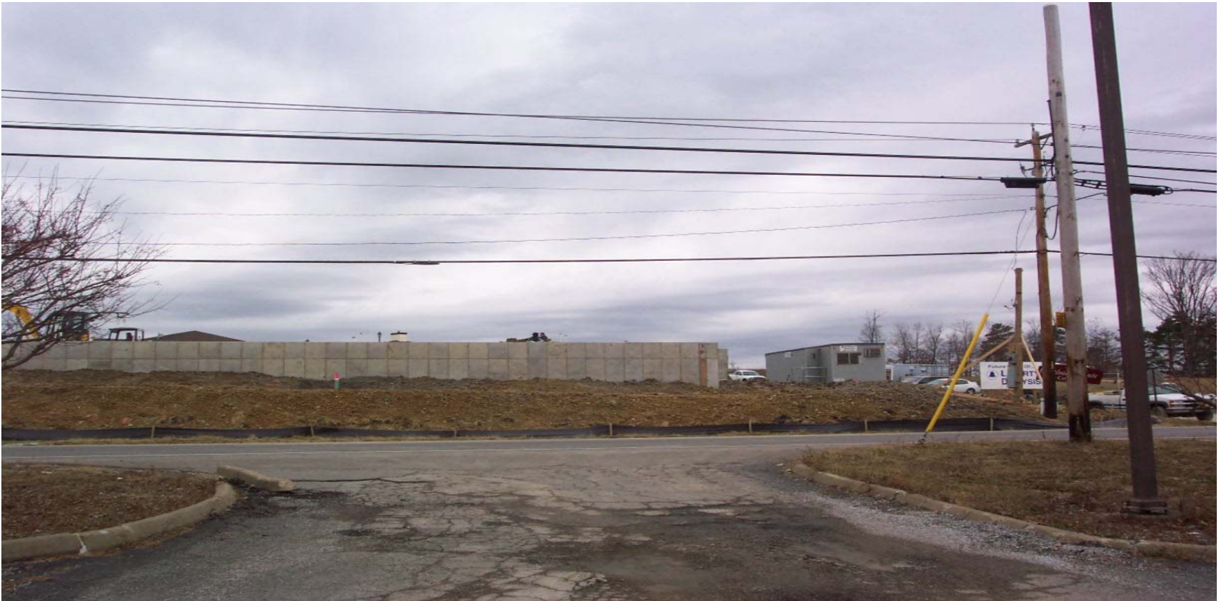
WPMA Medical Clinic LD under construction
