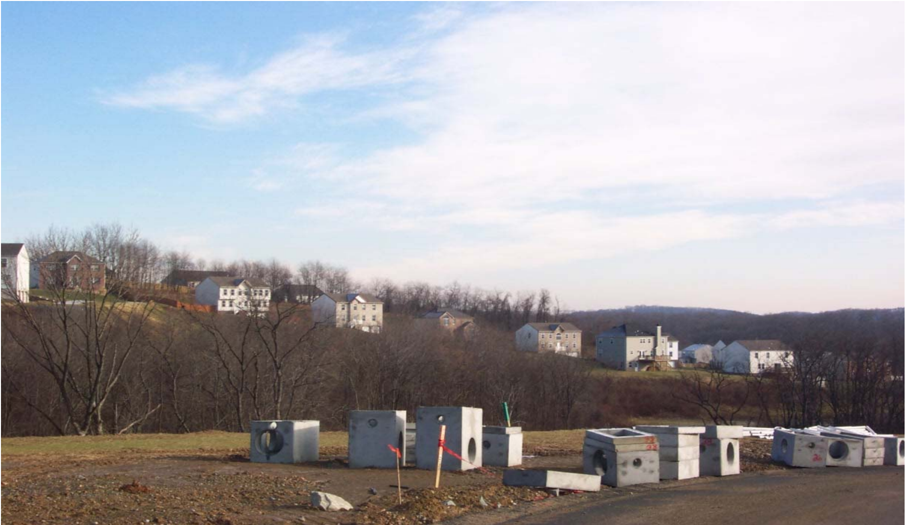
Whispering Pines Phase I completed, Phases II and III under construction
